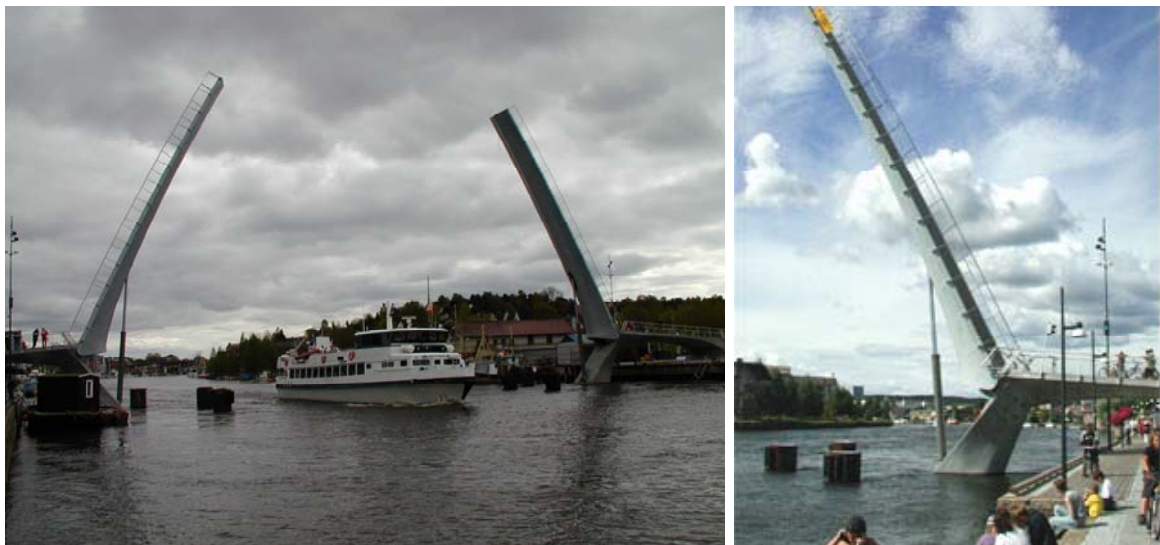
The bridge in open position
